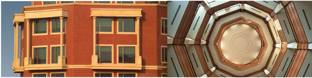
Fig. 5. Shading devices and central atrium of ITC Green Centre. Source: HPCB, 2010.
