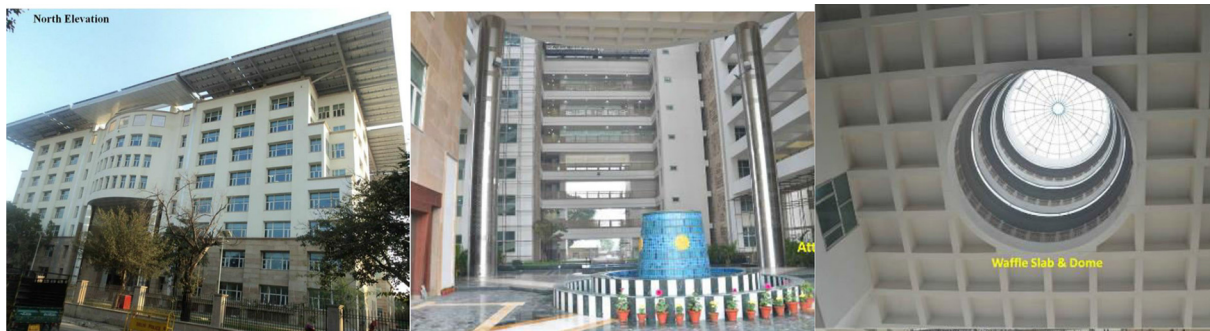
Fig. 12. North-side elevation and view of the central atrium of IPB. Source: Ministry of Environment and Forests, 2011.
