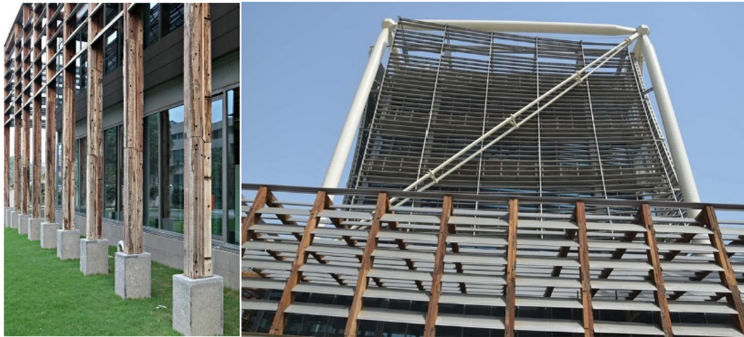
Fig. 11. Recycled wood used to clad columns and recycled railway sleepers used for making the louvers. Source: Singhal, 2014.
