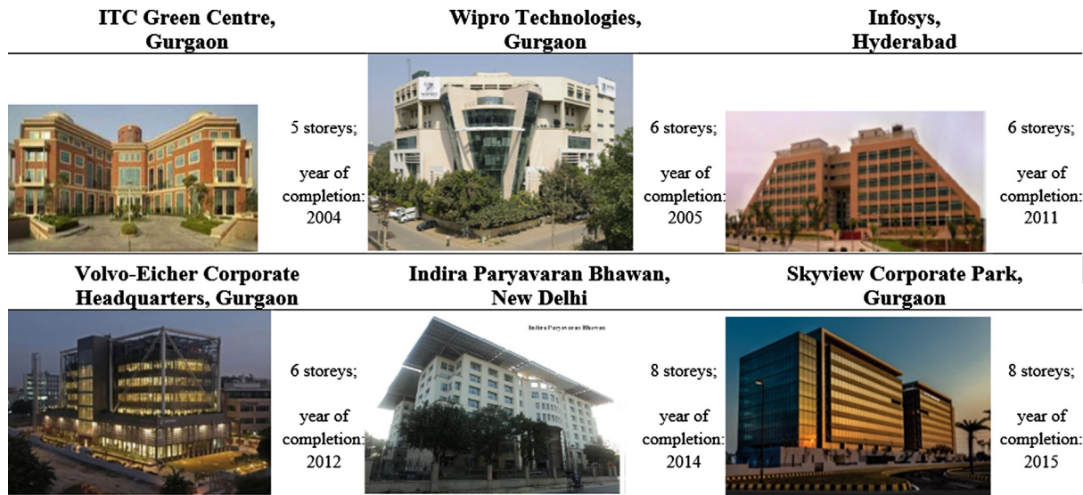
Fig. 3. Selected case studies of energy-efficient office buildings in composite climate. Source: Various.
